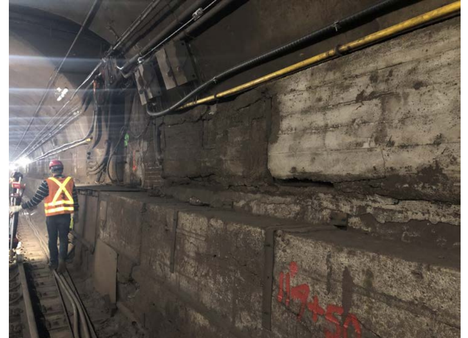
Bench wall in poor condition
