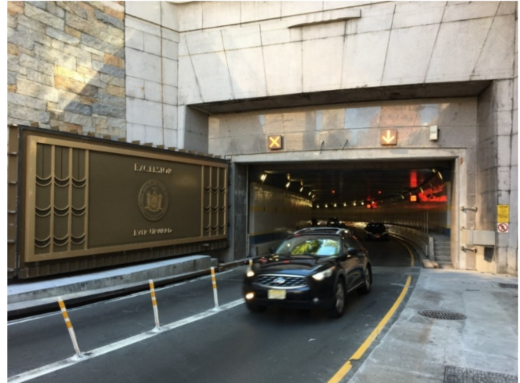
Watertight gate at Queens Midtown Tunnel
