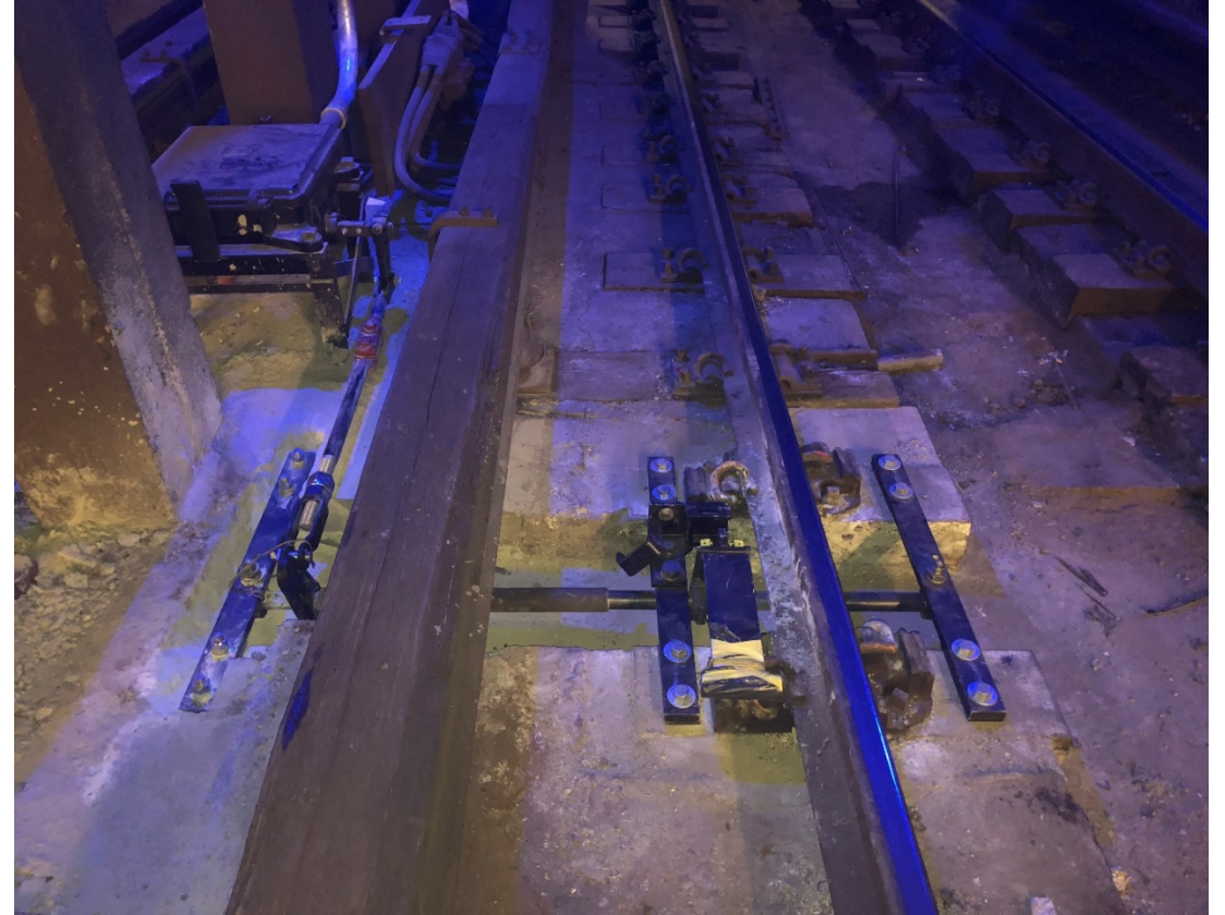
Installation of stop arm
